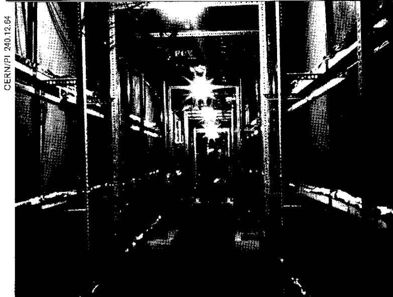
Physics underground. Photograph exhibited by Dr. Reines at the conference, showing part of a detection system for cosmic neutrinos installed at a depth of over 3000 metres in a mine in South Africa. The aim is to detect muons arising from neutrino interactions in the earth on either side. Tanks of liquid scintillator are arranged in two rows about 40 metres long and 2 metres high, each row having an upper, middle and lower section, so that some information can be obtained on the angle to the horizontal made by the muon path.
